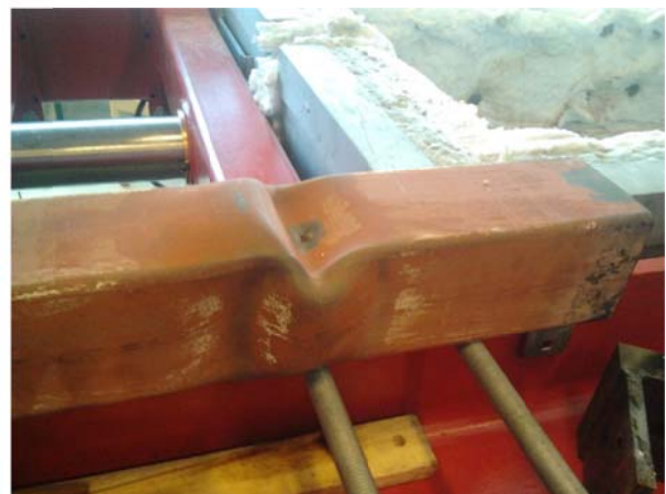
d) Steel SHS column damage.
